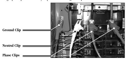
Single phase shown, third phase would require the third phase clip to be connected
