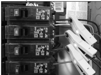
7. Plug CT clamp leads into the Transmitter. We recommend plugging each CT clamp into the output number that matches the actual breaker number. It is normal for the CT clamps to hum slightly due to magnetic fields caused by AC current. If there is considerable hum check to be sure all CT clamps are fully closed.
